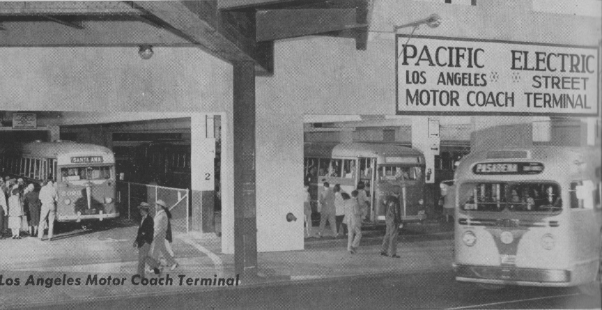
Sixth and Main Sts. Station
